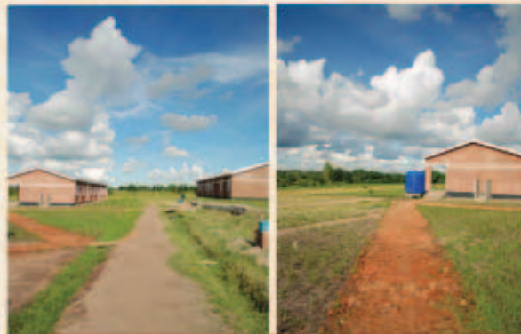
Construction of Pathways
