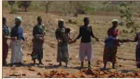
Women building the foundation on the first girls hostel
