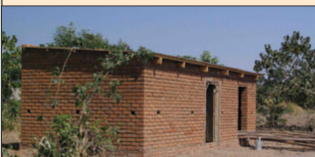
Storage Shed - our first completed building!
